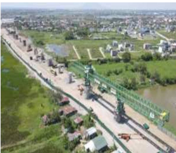
RAILWAY CONSTRUCTION. The launching gantry dubbed "Luid" used in the construction of the North-South Commuter Railway (NSCR) Malolos-Clark segment in this undated photo. Acting Transportation Secretary Giovanni Lopez said Thursday (May 28, 2026) that more than 31,000 jobs for Filipinos have been generated by the NSCR and the Metro Manila Subway Project. (Photo courtesy of DOTr)
