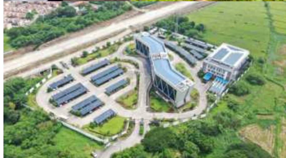
Aerial view of the MPT South Hub, featuring 1,184 solar panels that generate about 97% of the building's energy needs. The facility also has a rainwater harvesting system that reduces water use by 10%, along with EV charging stations for company electric vehicles.
